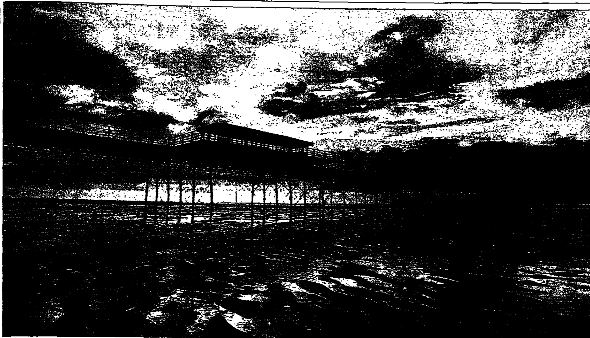
RUST and rot are threatening Southport Pier (above), the second longest in Britain and the inspiration for dozens of Victorian cast-iron seaside fantasies. Writes Maryn Halsall. The Grade II listed structure, which heralded the high watermark of seaside pier construction, faces demolition without significant lottery funding.
